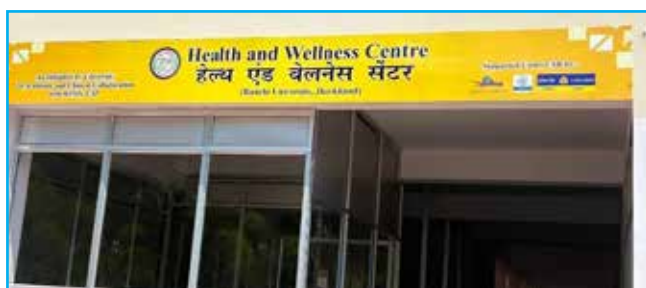
Supported for repair and renovation of Wellness centre of Ranchi University, Jharkhand
