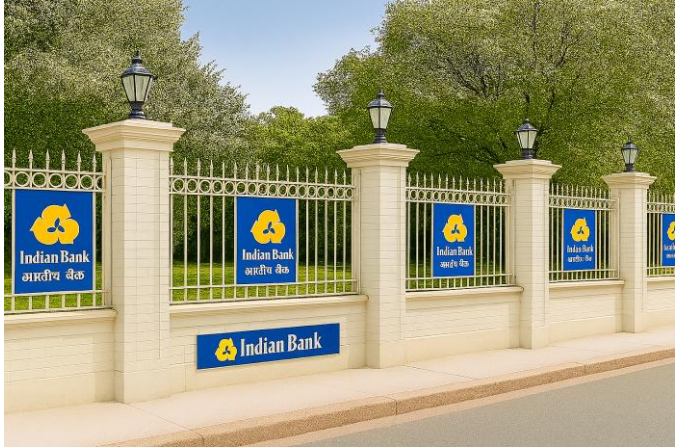
BOUNDARY WALL VIEW
